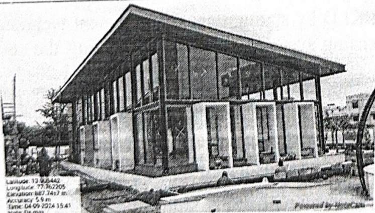
Partly civil & metal structure at Southern side of the apartment
